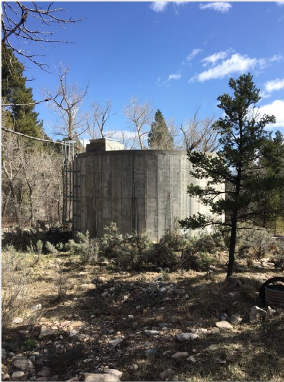
Image 6 – 0.1-million-gallon Upper Concrete Tank
