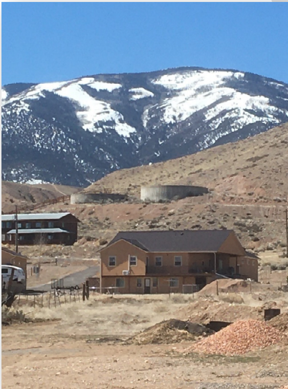
Image 4 – 0.20 and 0.15 million Gallon Lower Concrete Tanks
