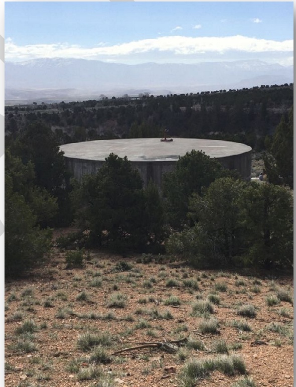
Image 5 - 0.25-million-gallon Middle Concrete Tank
