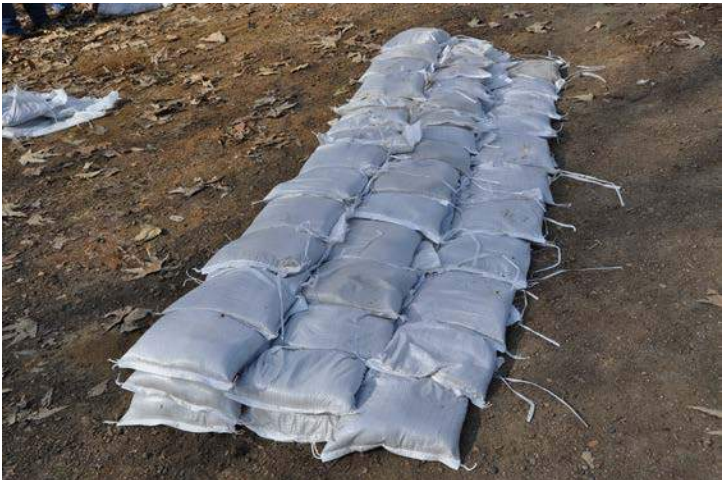
Sandbag Wall Construction
